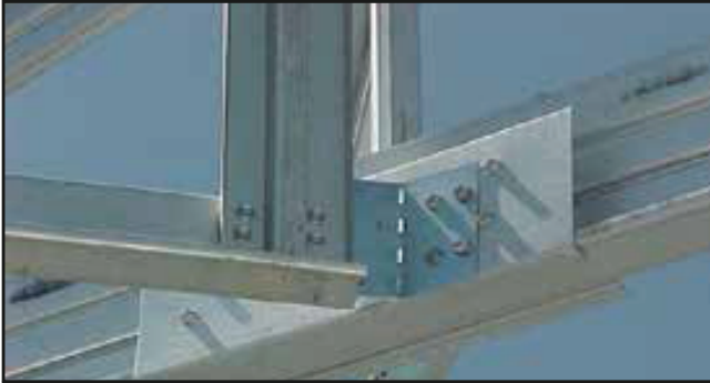
TRUSS TO TRUSS CONNECTIONS
