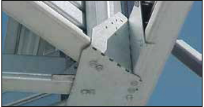
TRUSS TO TRUSS CONNECTIONS
