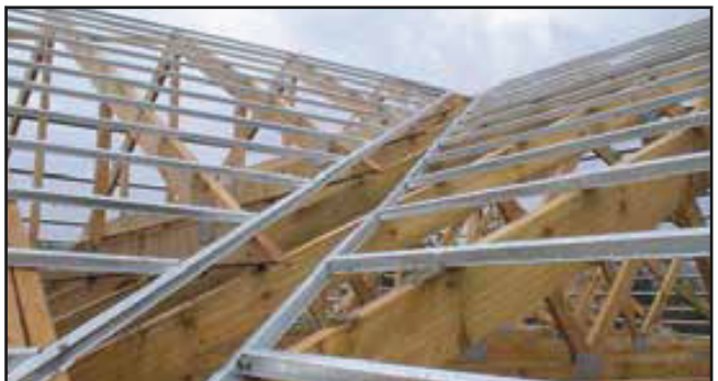
STEEL PURLINS ON TIMBER ROOF
