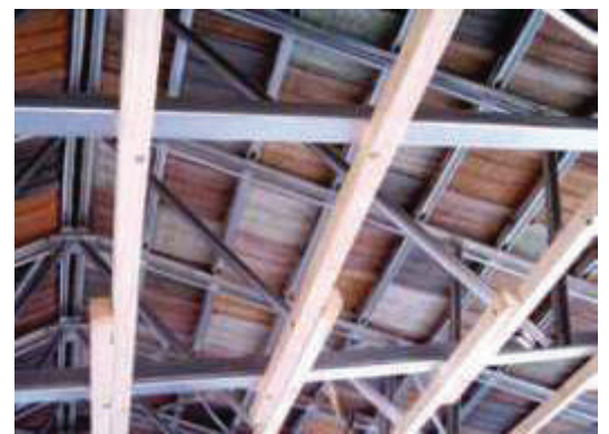
STEEL PURLINS ON TIMBER ROOF
