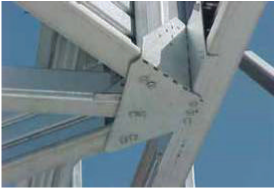
TRUSS TO TRUSS CONNECTIONS
