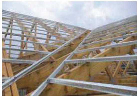
STEEL PURLINS ON TIMBER ROOF
